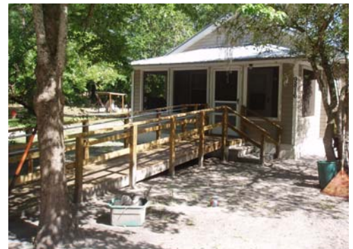
Home Repair Program: Wheelchair Ramp built
